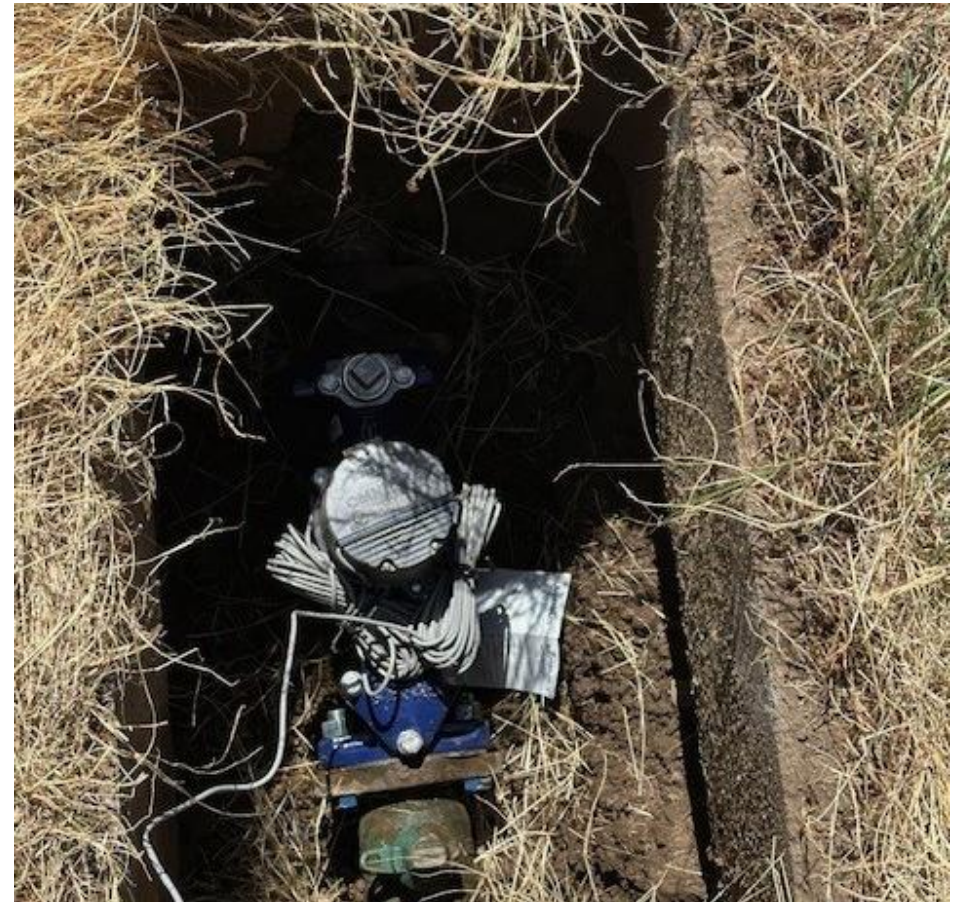
Replaced Water Meter at 2700 Portland Road (Newberg Chevrolet)
