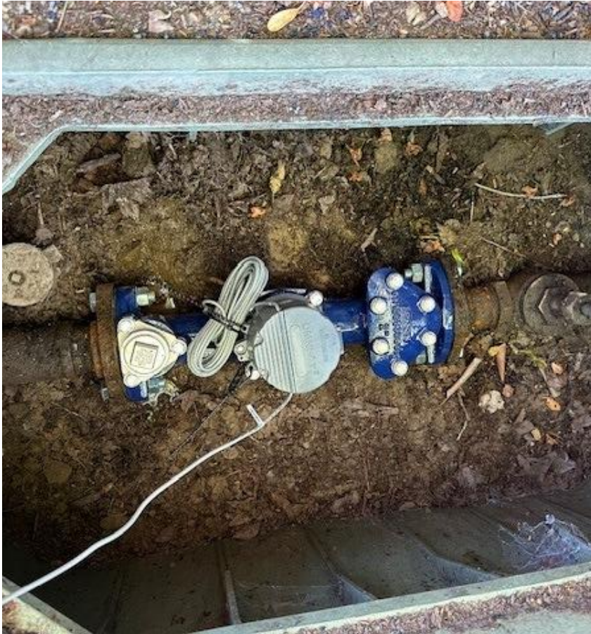
Replaced 2" meter at George Fox University
